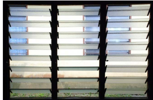
Figure 6: Frosted Glass Louvered Windows
