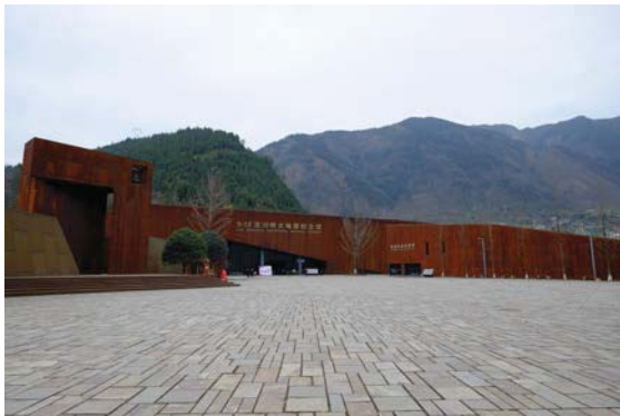
Figure 13. The plaza of memorial and the entrance of the memorial
