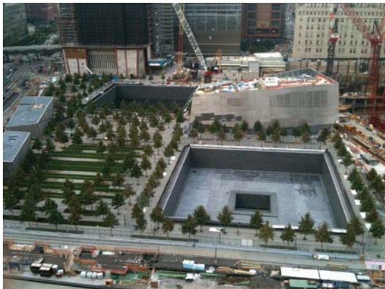
Figure 20. Two huge holes left by the collapse of World Trade Center be transformed into memorial named “Reflecting Absence”
