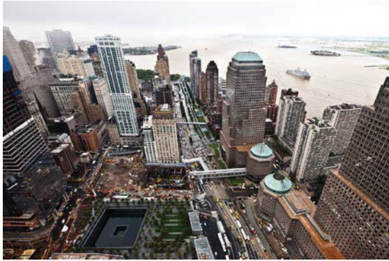
Figure 19. The Site of World Trade Center is extremely complex
