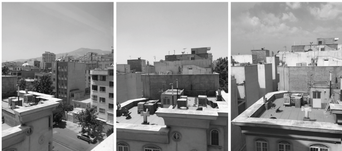
Figure 1. A Typical Visual Appearance of Urban Neighborhoods in Tehran City with Viewpoints to the Current Rooftops of Mid-Rise Residential Buildings
