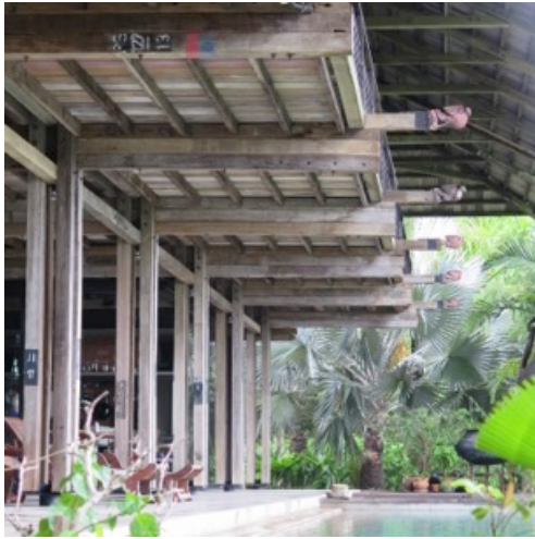
The Telegraph Pole House, Langkawi (Photograph by author)
