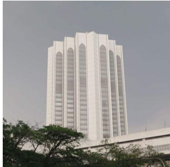
The Dayabumi Building (Photograph by author)
