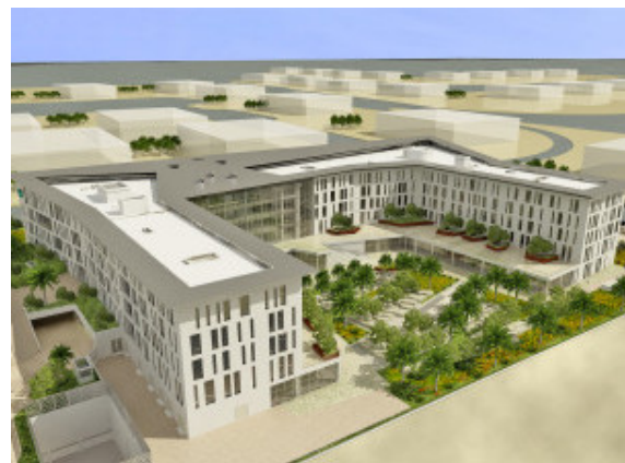
Figure 3: Credit Agricole Egypt New Head Office
