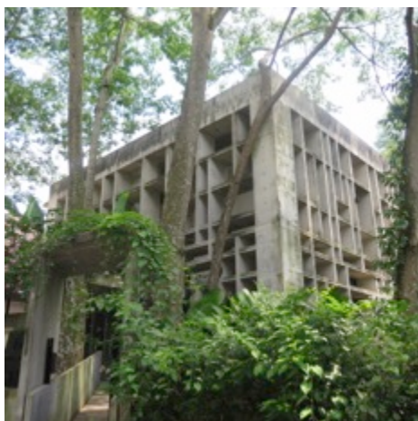
The Chempenai House (Photograph by author).
